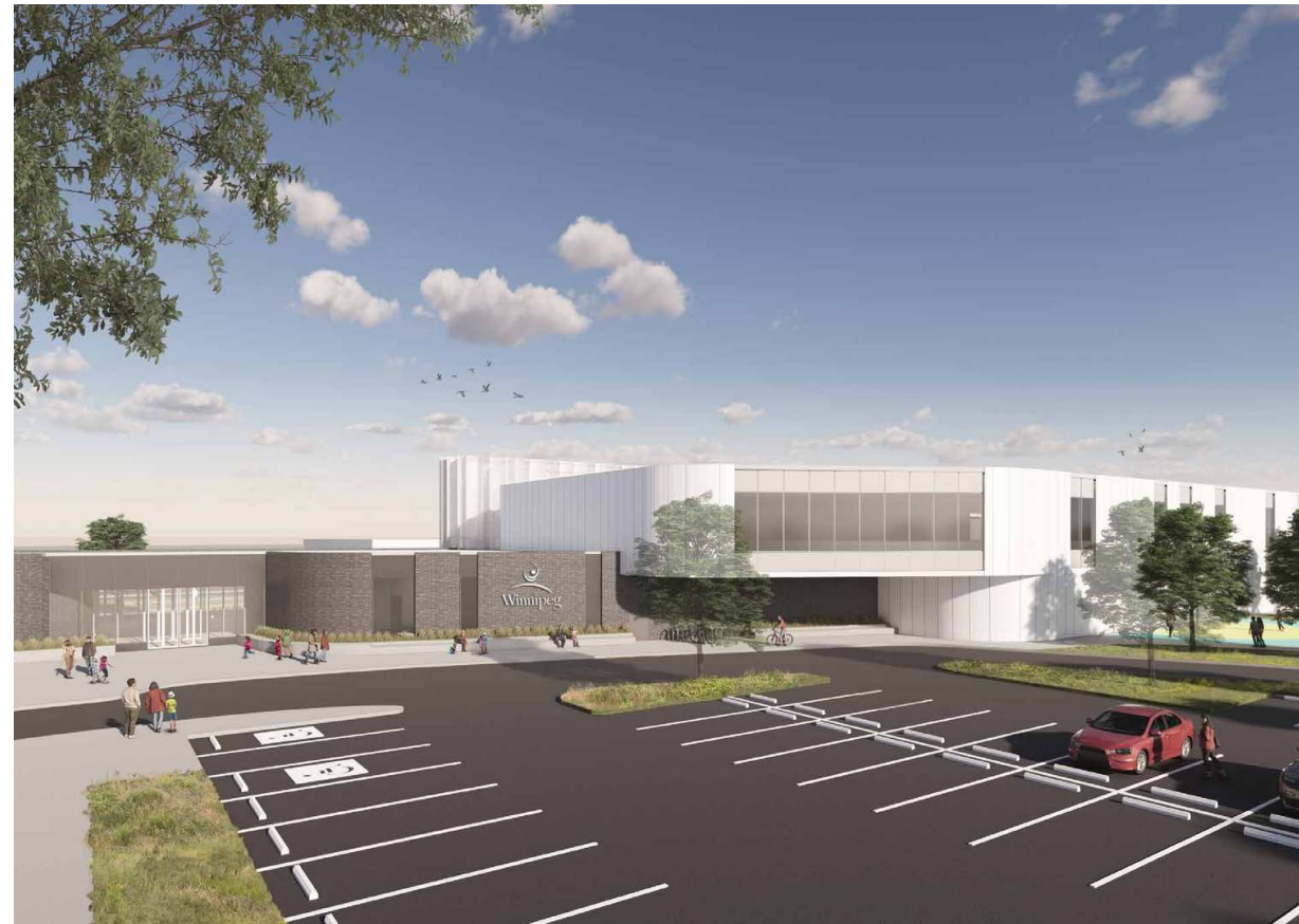
Exterior daytime view (looking south-west).
