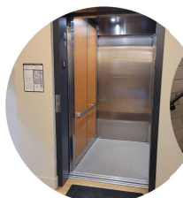
New addition: elevator
