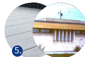
5. New roofing & wood screen
