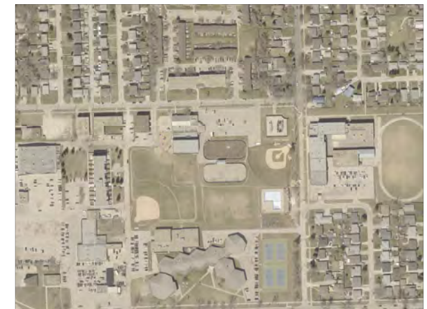
Winakwa Community Centre
