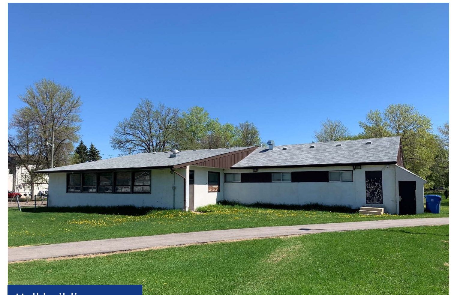
Hall building - rear
