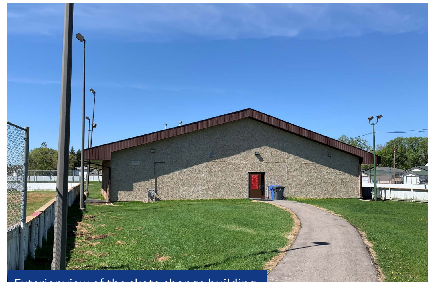
Exterior view of the skate change building
