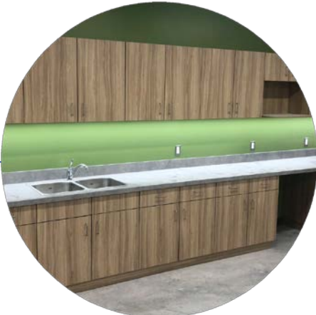
Accessible kitchenettes & closets
