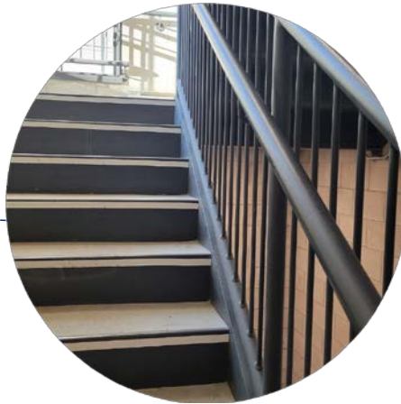
Stair safety upgrades
