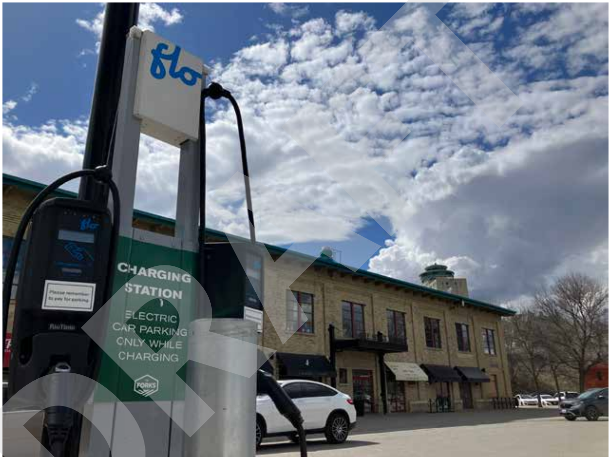
Electric Vehicle charging station at The Forks.
