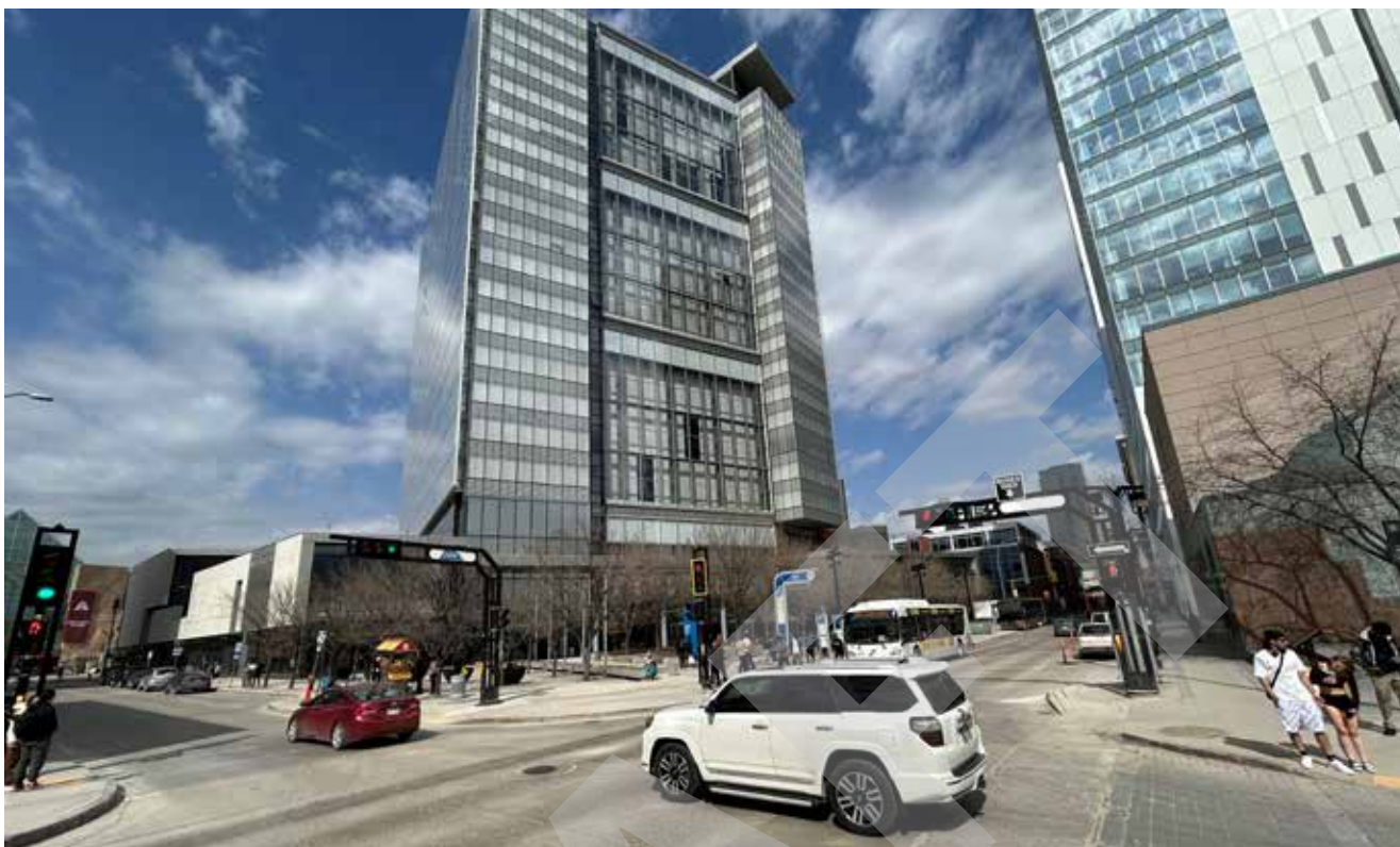
Graham Avenue at Edmonton Street (Manitoba Hydro) today (looking east).
