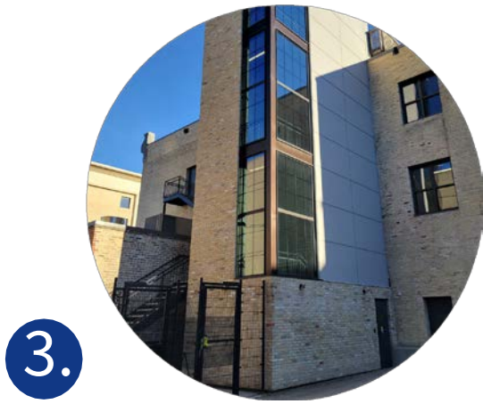
Elevator & stair addition
