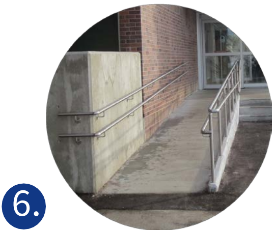
New concrete landings & ramp
