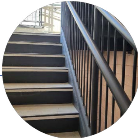
Stair safety upgrades
